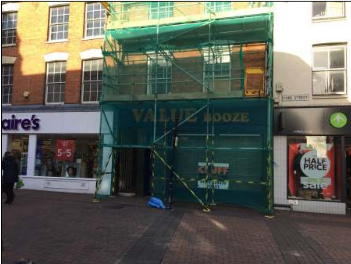
(Scaffolding in place due to works being carried out to the upper floors).
